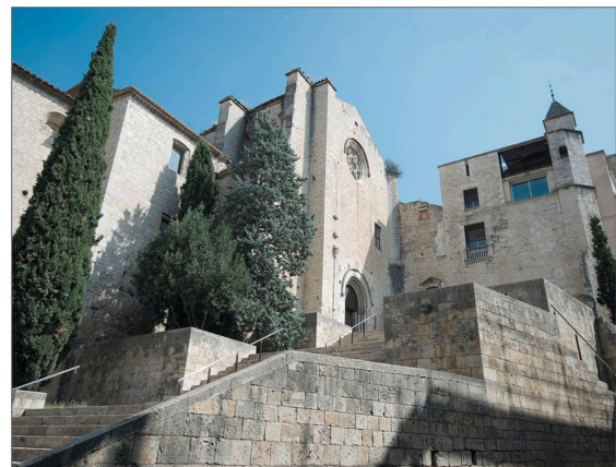
Main entrance to Aula Magna
